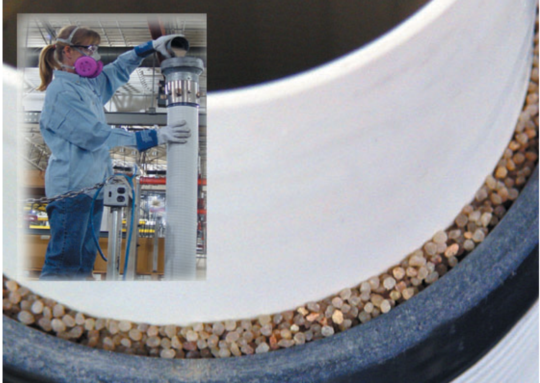
Carefully placed filter pack is 100% void-free.
